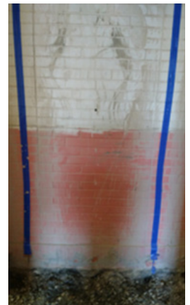
Future doorway in Girls' Restroom
