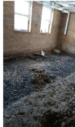
Boys' Restroom, Floors Removed
